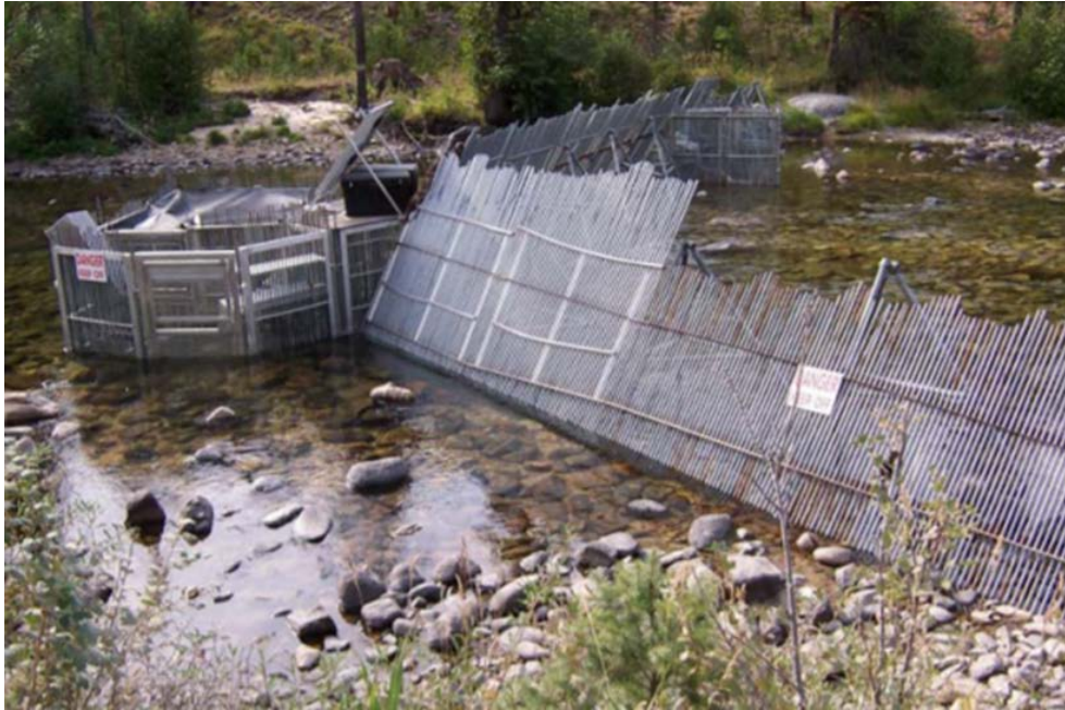
Figure 5-4. Upstream and Downstream Trap Box Currently Used in Johnson Creek
