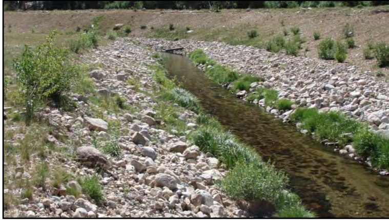
Photo 3-3. Rock-Lined Reach of Meadow Creek Around the SODA.
