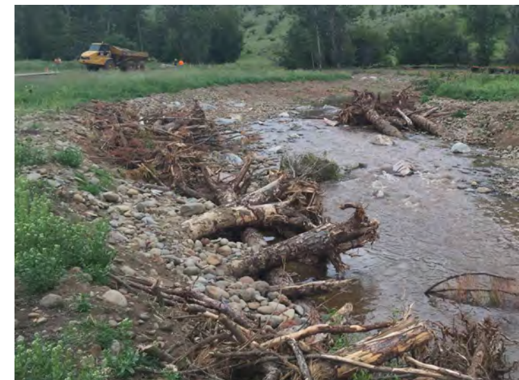
EXAMPLE: INSTALLED TOE LOG STRUCTURE (FOREGROUND)
