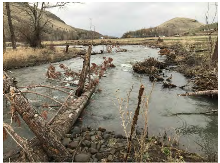
EXAMPLE: INSTALLED TYPICAL SWEEPER LOG STRUCTURE
