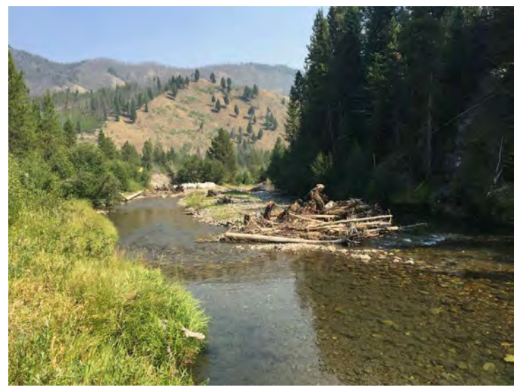
EXAMPLE: INSTALLED APEX LOG STRUCTURE
