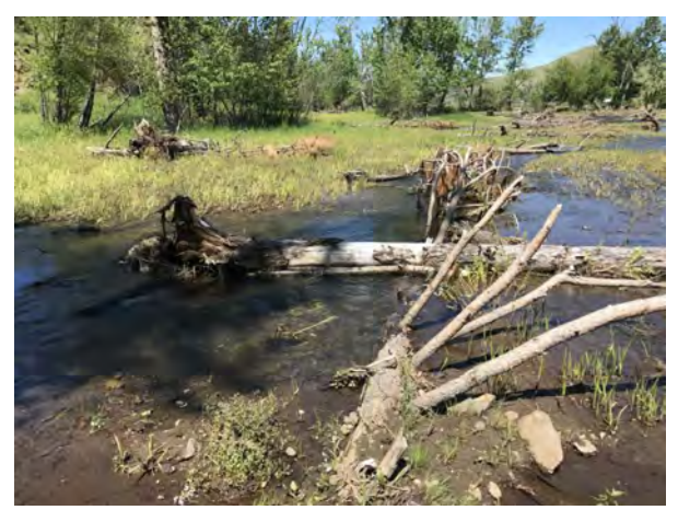
EXAMPLE: INSTALLED LOG FLOODPLAIN ROUGHNESS STRUCTURE
