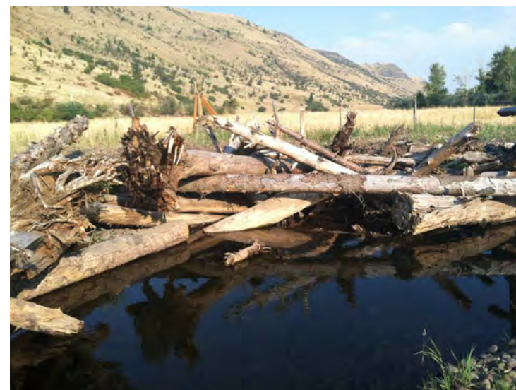
EXAMPLE: INSTALLED TIGHT RADIUS JAM STRUCTURE
