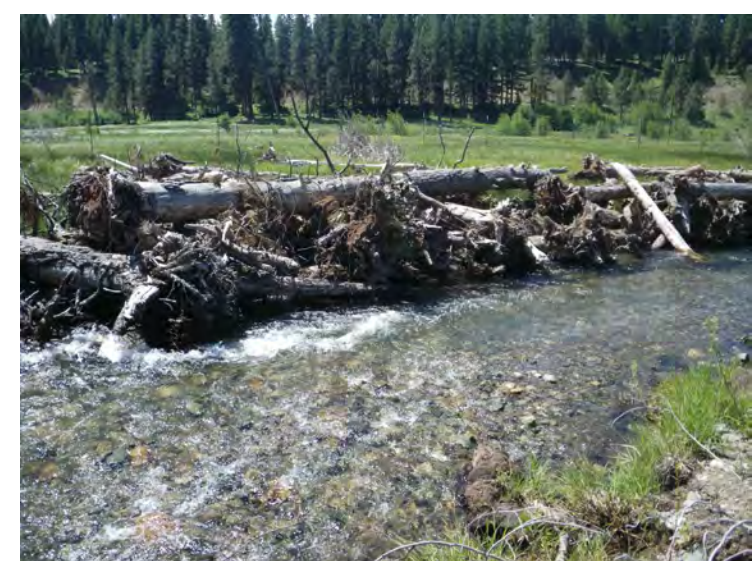
EXAMPLE: INSTALLED BEND JAM STRUCTURE
