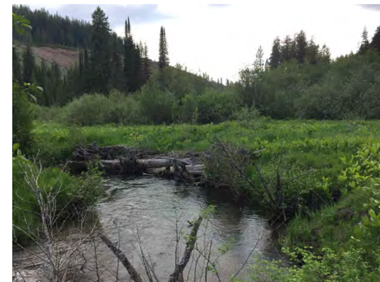
EXAMPLE: INSTALLED TIGHT RADIUS JAM STRUCTURE
