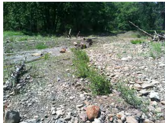
EXAMPLE: INSTALLED LIVE WILLOW TRENCH
