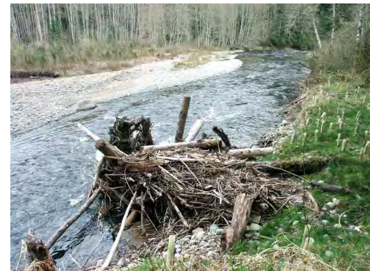
EXAMPLE: INSTALLED TOE LOG STRUCTURE
